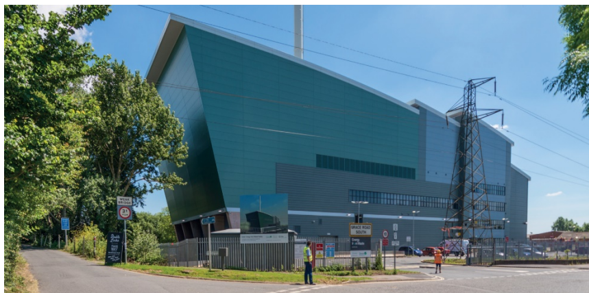
Figure 23: Exeter Energy Recovery Facility
